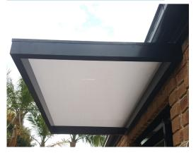
Frame Size: 150mm Welded Aluminium Box
