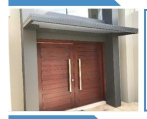
Frame Size: 100mm Welded Aluminium Box
