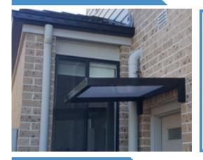
Frame Size: 50mm Welded Aluminium Box
